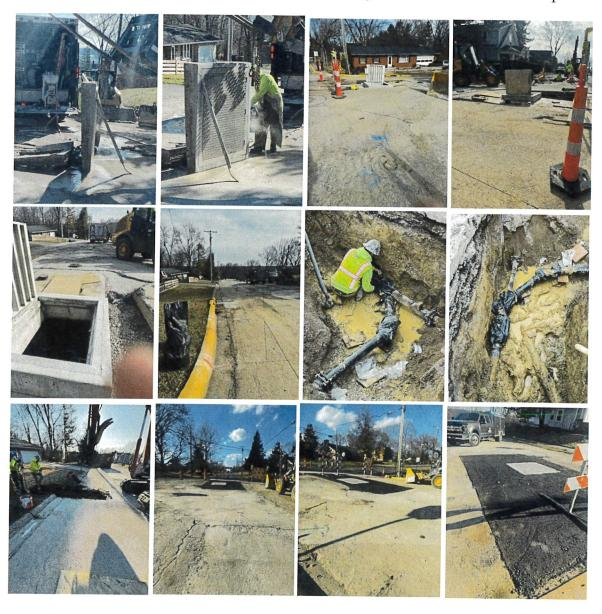
• I am providing a Third Street waterline and storm waterline update. Smith Corp has completed the waterline from High Street to Franklin Road. They are taking bacterial samples and doing pressure tests on the main waterline. They will start the lateral lines upon approval of all the tests.
